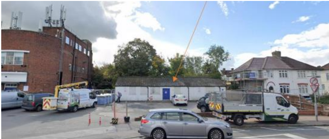
Figure 5: Existing Outbuilding will be demolished
