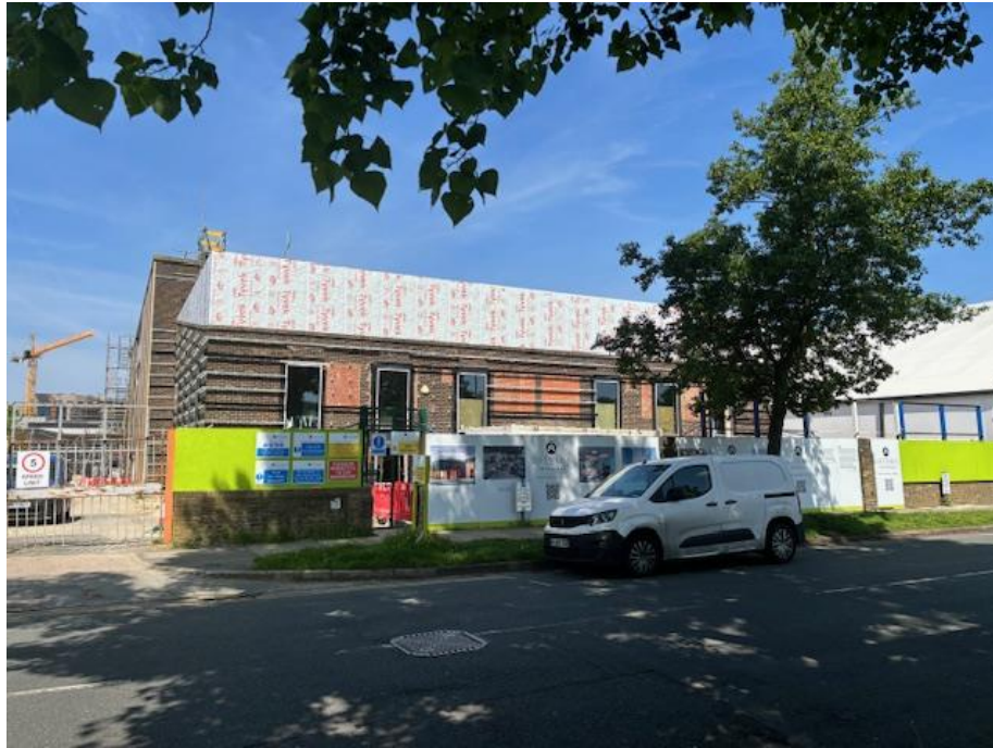
Figure 3 – Front elevation facing Copers Cope Road (13/05/24)
