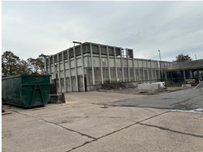
Figure 10 – existing cladding and walls (tanks to be sited adjacent)
