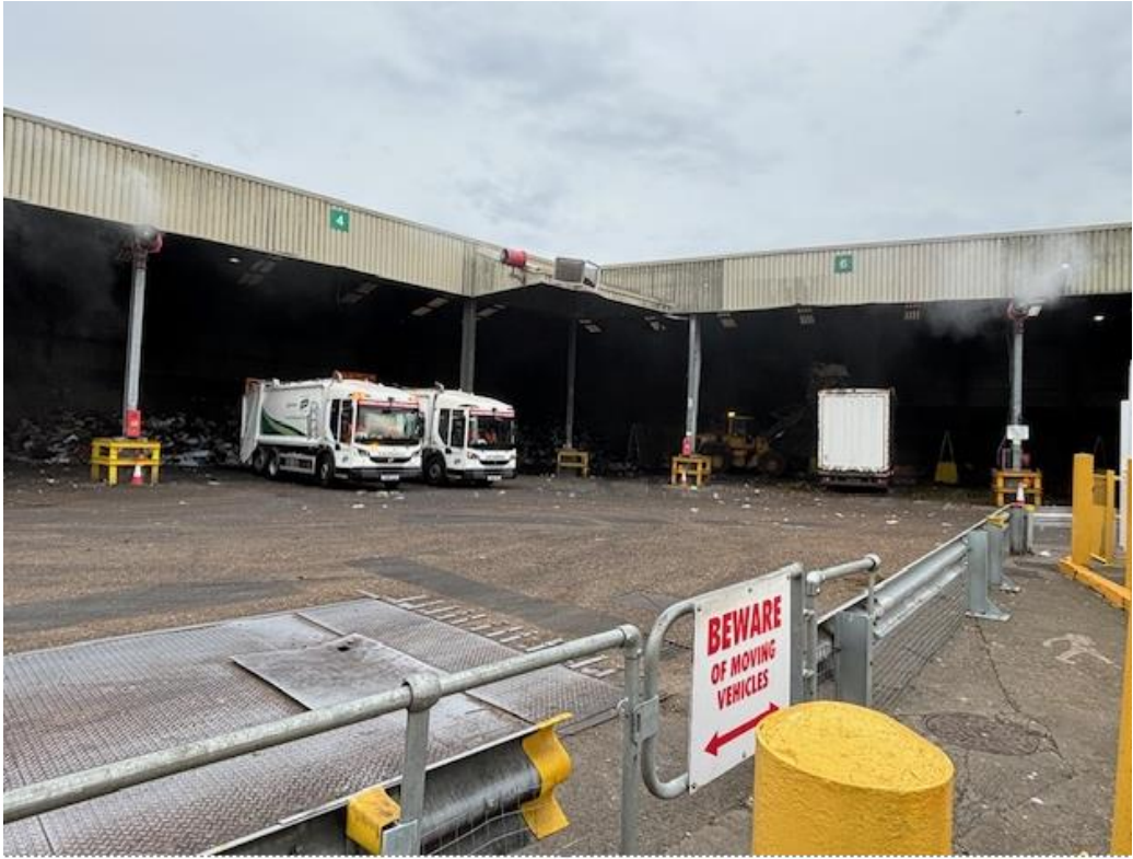
Figure 8 – Facing north east
